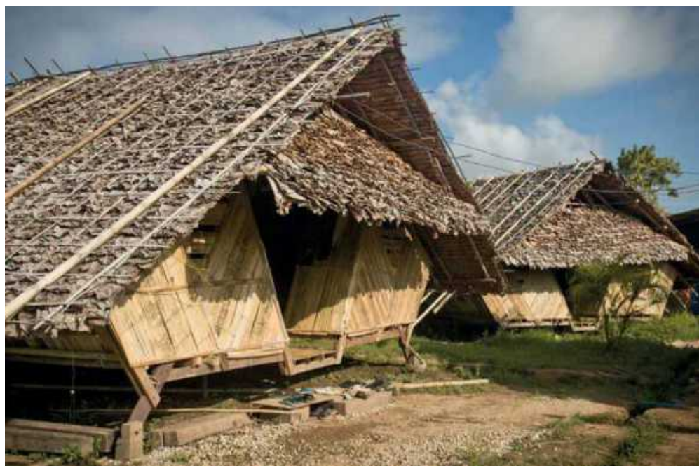
Courtesy Bamboo Temporary Dormitories © F. Pallarès López
